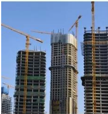
Engineering tower crane
